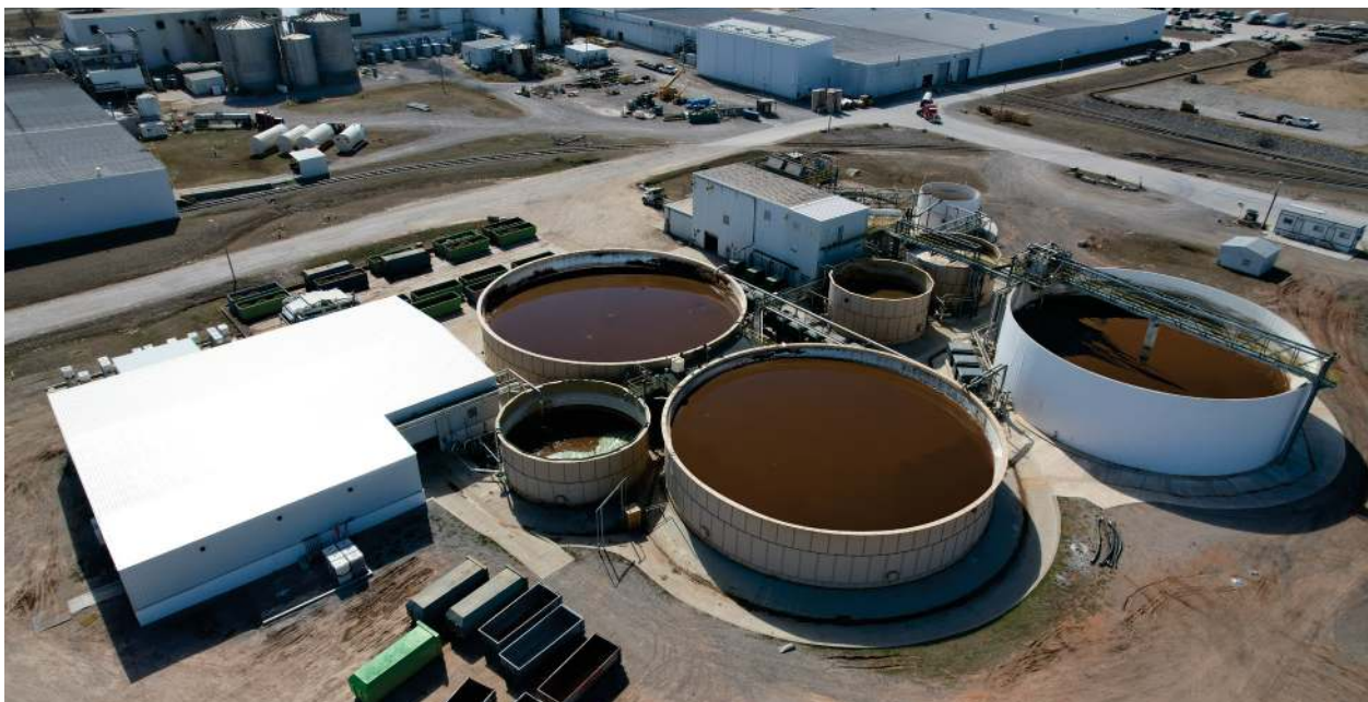
New water treatment facility at Republic Paperboard in Lawton, OK.
